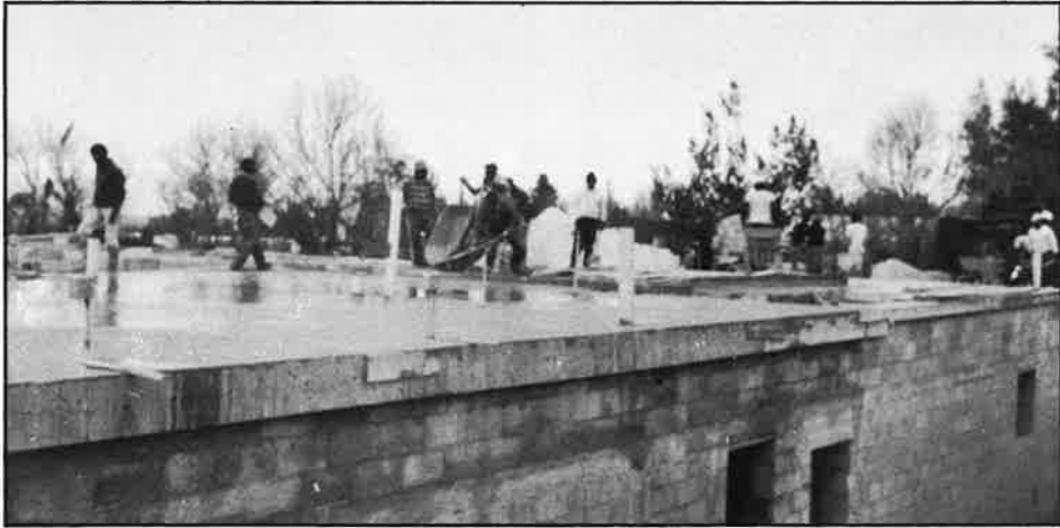
Completion of Second Floor.
